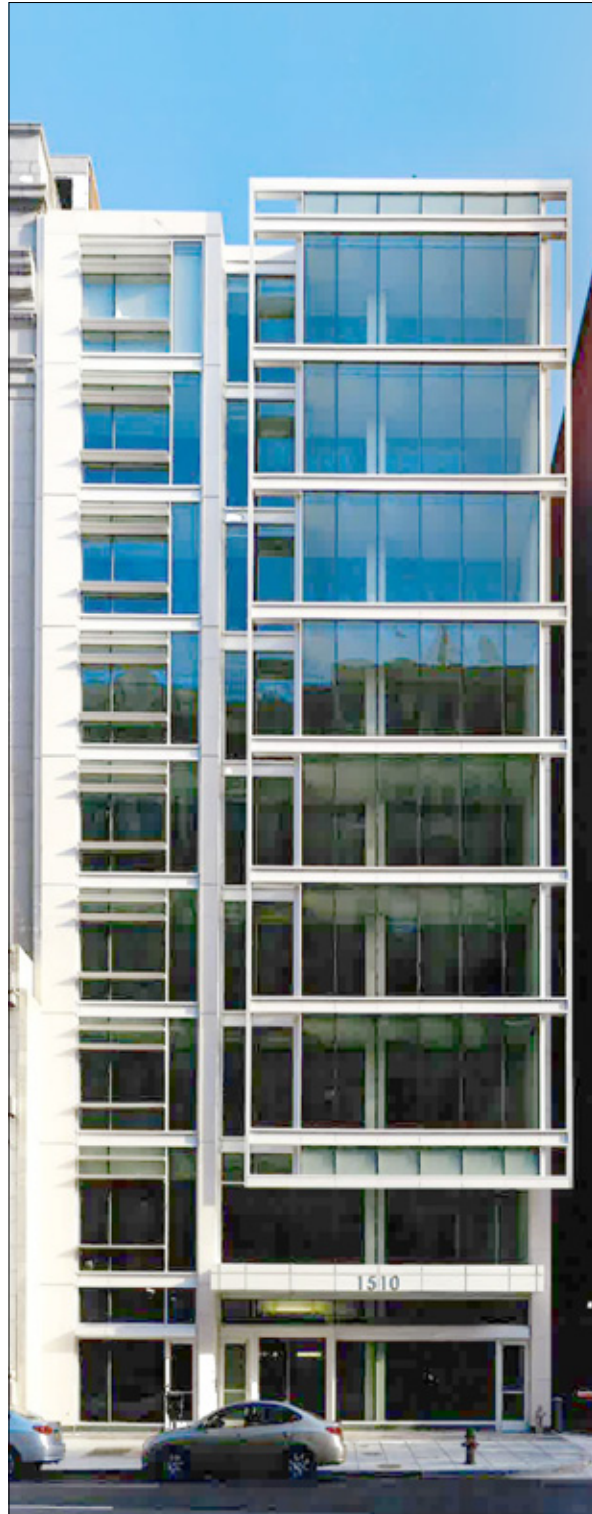
TCA's Washington office at 1510 H Street, NW, near the White House and Lafayette Park.
